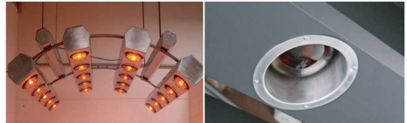
Cooling fan for each row of lights
